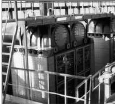
Fig 23. UV drinking water plant 405.000 m 3 per day, Tolmazyti (Russia)
